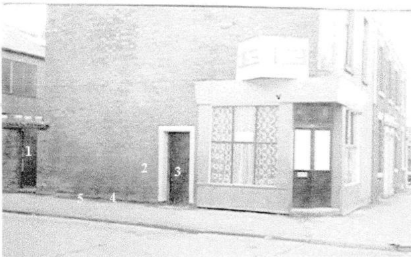
The 3 DOORS in ELLEN STREET. 1: yard door. 2: blocked doorway. 3: cellar door leading to bakehouse. 4: coke shute. 5: window -now paved over.
