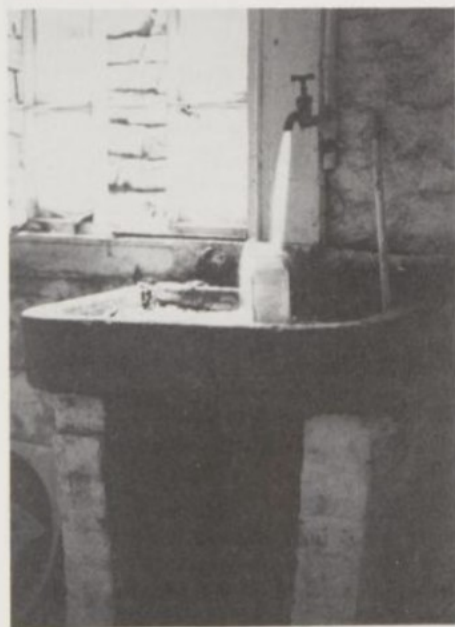
Fig. 14: Tap and slopstone, c.1840, Cross Street.
