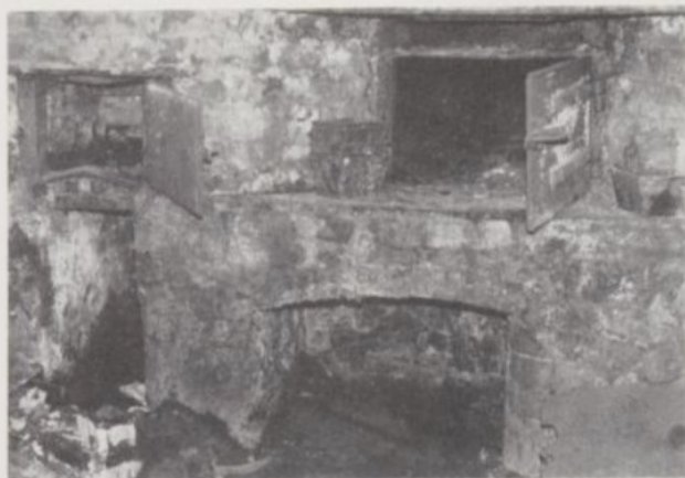
Fig. 69: Bread oven in cellar bakehouse at No.40 Brackenbury Street (demolished 1982).
